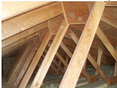
Interior view of attic
