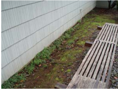
Drainage directed towards front of building
