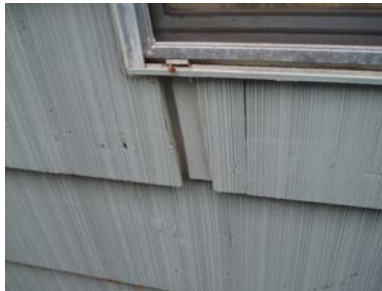
Example of deteriorated siding at rear
