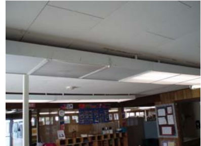
Example of damaged fixture
