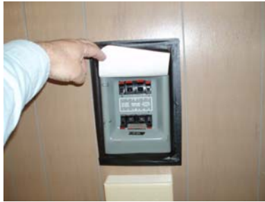
FPE Stab-Lok panel
