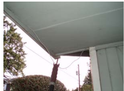
Example of deterioration at soffit
