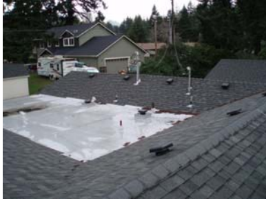
Low pitched, single-ply roof
