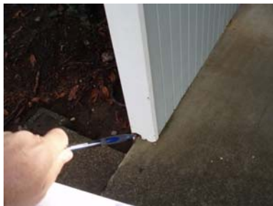
Example of deteriorated trim
