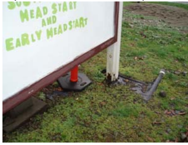
Example of deteriorated sign post
