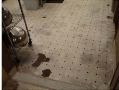
Example of staining/damage at flooring
