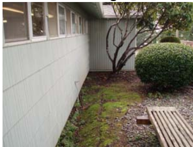
Eroded line on ground sign of overflowing gutter
