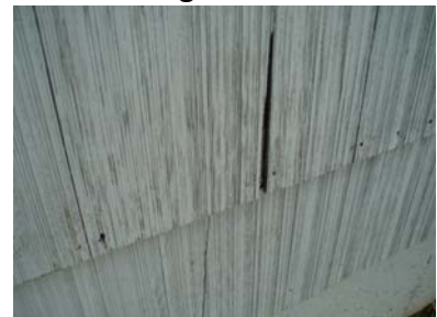
Example of deteriorated siding at right side
