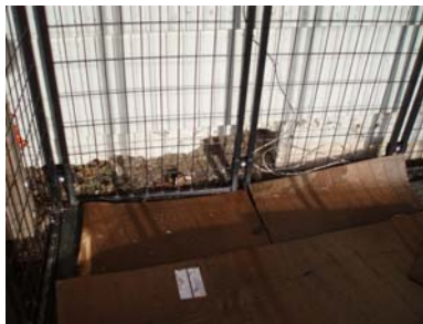
Erosion or undermining at slab
