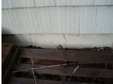
Example of common concrete crack
