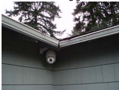
Example of damaged gutter/leaking seam
