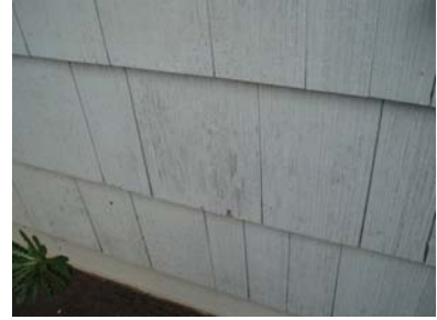
Example of deteriorated paint
