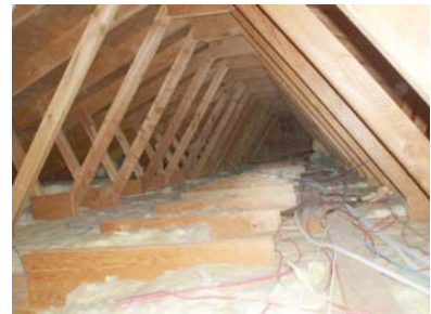
Interior view of attic
