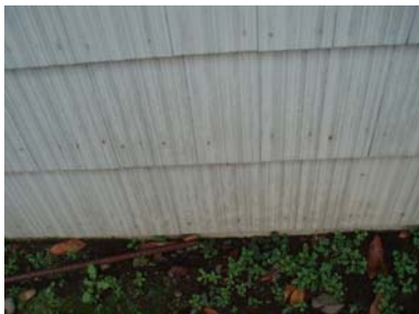
Example of corroded fasteners
