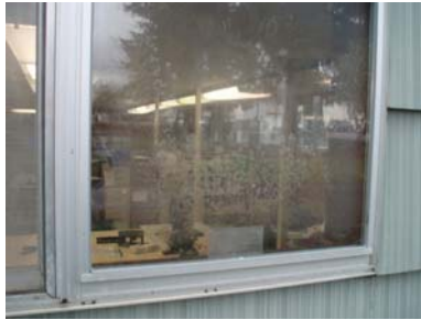
Example of staining between panes
