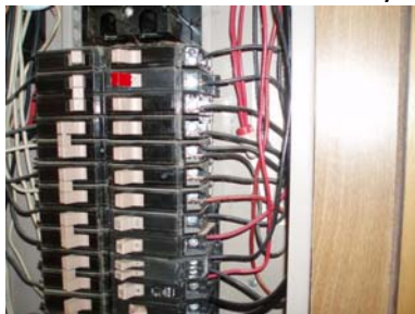
Two wires connected to 5 th breaker from top
