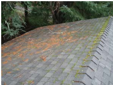
Moss and debris on roof
