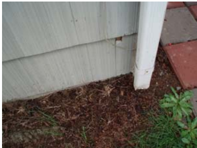
Example of damaged siding at rear
