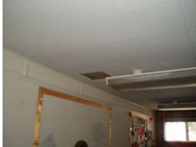
Example of missing ceiling tile
