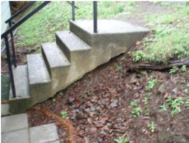
Erosion under steps
