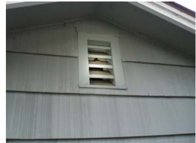
Damaged vent screen
