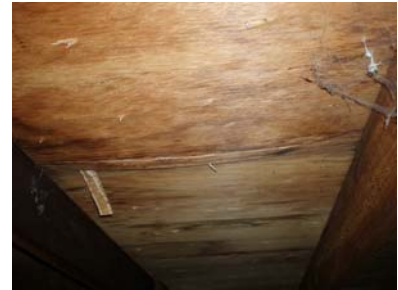
Damaged area of roof decking
