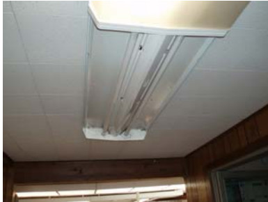
Example of missing bulbs
