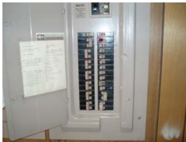
Double pole circuits at left marked "DO NOT USE"
