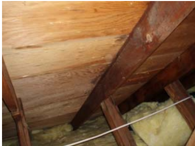
Example of staining at roof decking
