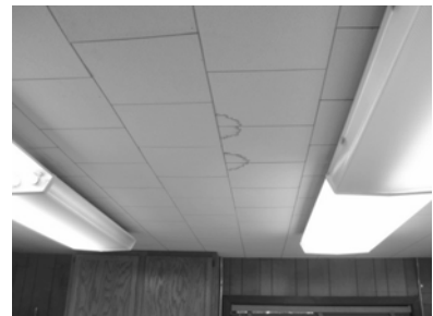
Example of ceiling stains
