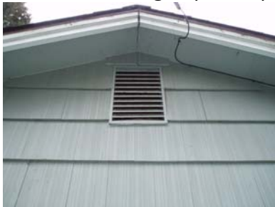
Damaged vent screen
