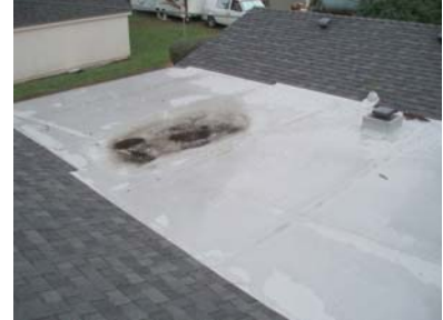
Area of ponding
