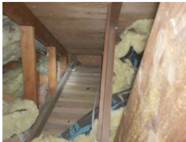
Example of missing insulation
