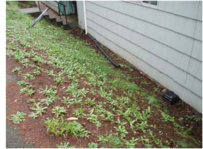
Drainage directed towards left side of building
