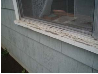
Example of deteriorated paint
