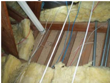
Example of missing insulation
