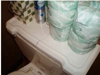
Cracked toilet tank lid at staff bathroom
