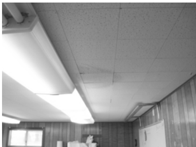
Example of ceiling stains
