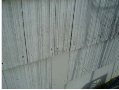
Example of siding repair area
