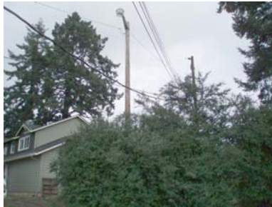
Electric service passing through trees
