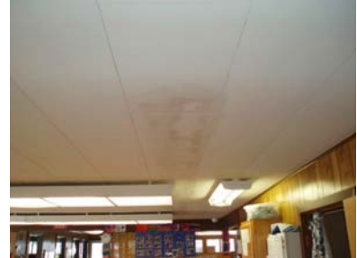
Example of ceiling stains
