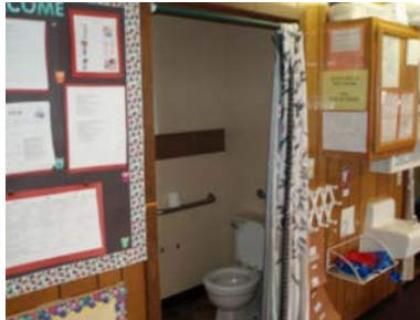
No door at bathroom
