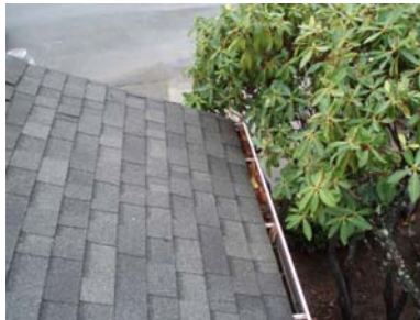
Debris in gutters
