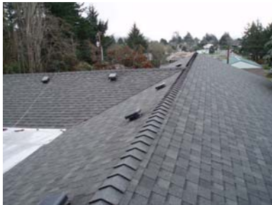
General roof view
