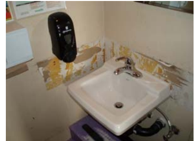
Sink loose on wall
