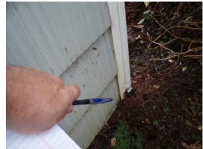
Example of deteriorated siding where in contact with ground
