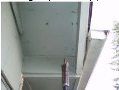
Example of deterioration at eave
