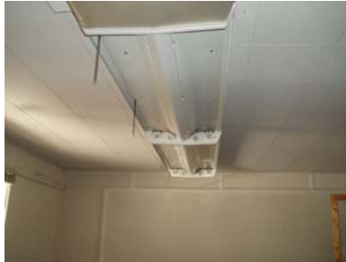
Example of missing bulbs/covers
