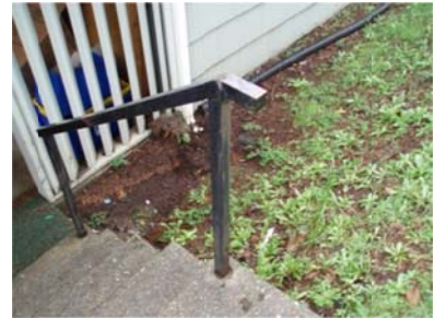
Example of handrail extending beyond post
