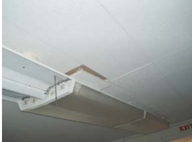
Example of damaged ceiling tile
