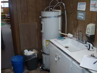
Water heater TPRV drains to sink
