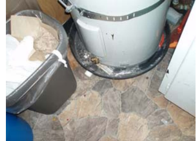
Drip pan drains to floor
