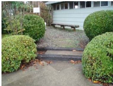
Uneven steps at approach to seating area
